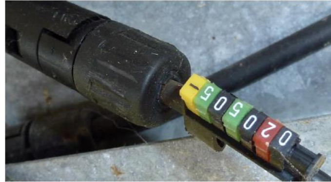
Fig. 4-14: string connector on negative pole of string 0205-05
