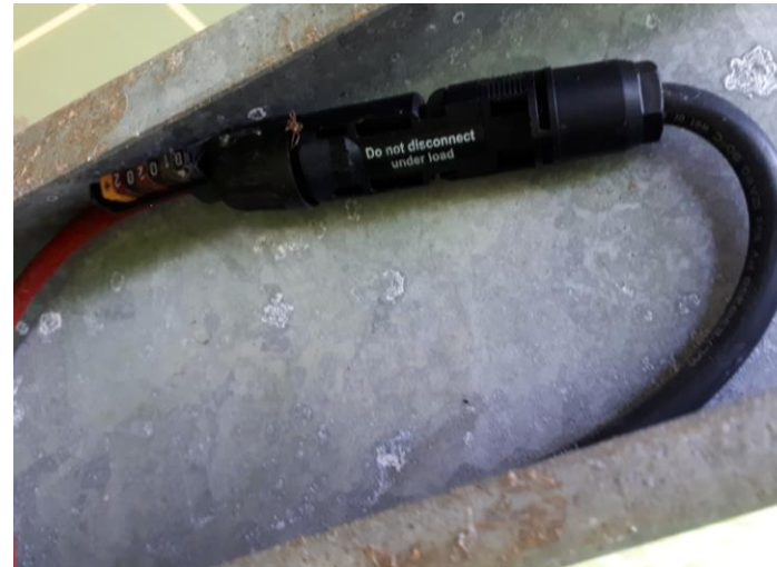
Fig. 4-14: string connector on negative pole of string 0205-05
