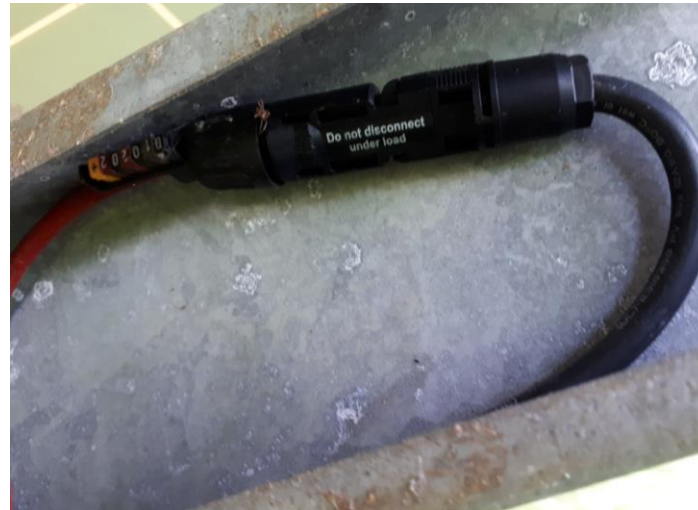
Fig. 4-14: string connector on negative pole of string 0205-05
