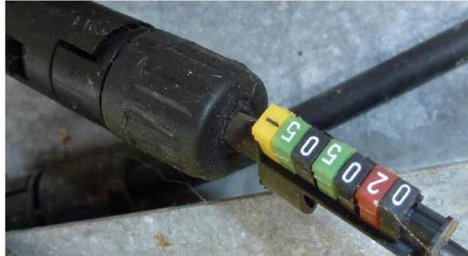
Fig. 4-14: string connector on negative pole of string 0205-05
